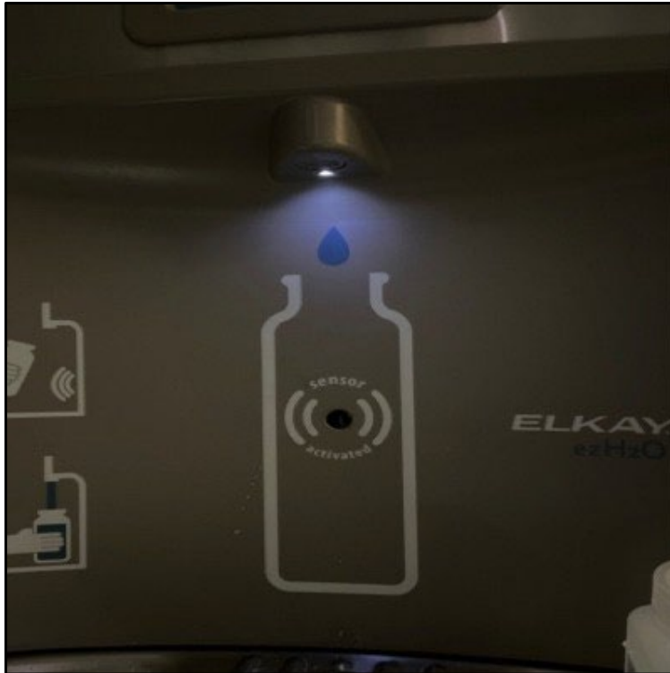
View of potential DWO and sample 03-02-00H-DW-P-18
