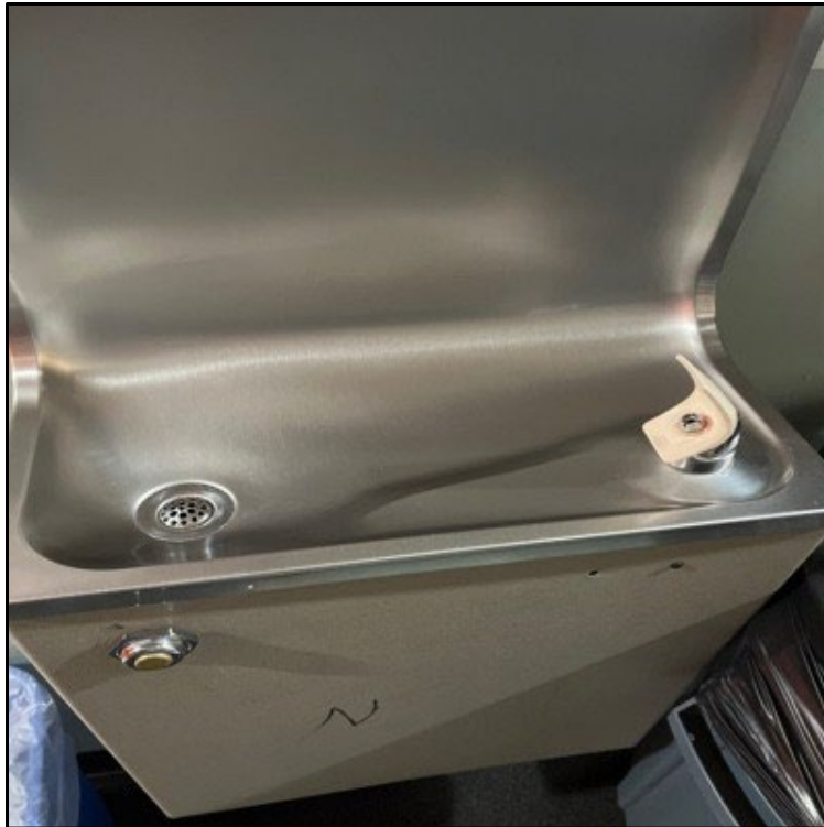
View of potential DWO and sample 03-01-00H-DW-P-3
