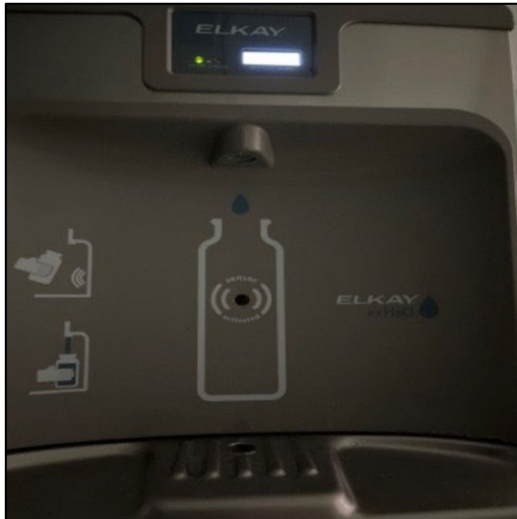
View of potential DWO and sample 03-01-00H-DW-P-7
