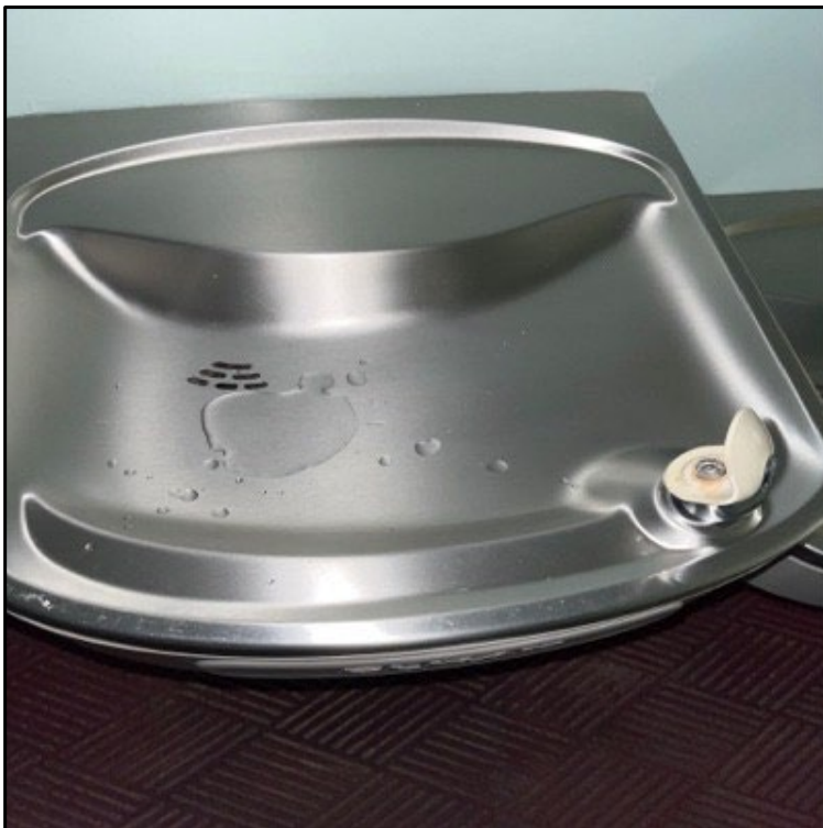
View of potential DWO and sample 03-01-00H-DW-P-10
